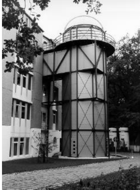
Figure 4.1-5 Building for the new SLR station at GFZ Potsdam. The laser transmitter is located inside the tower below the dome's platform whereas the control and measuring electronics is contained in a laboratory of the neighboring main building.
