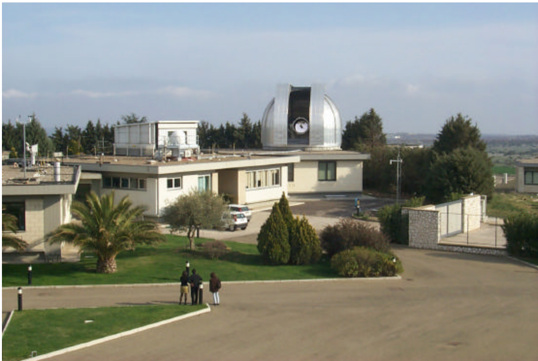
Figure 4.1-2 shows the 1.5 meter MLRO telescope through the slit of the 9.5 meter dome. The aircraft detection radar's white dome is visible on the roof of the old SLR system.
