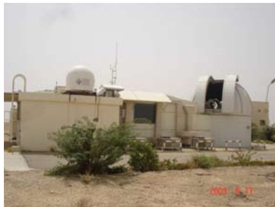
Figure 13-63. SALRO today with aircraft radar and air-conditioning system upgrade.
