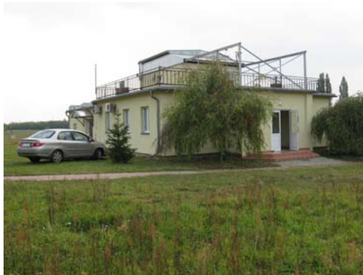
Figure 13-8. The Borowiec SLR building after renovation
