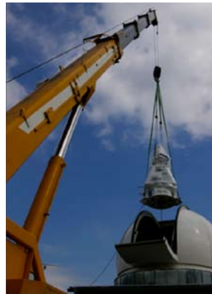
Figure 13-81: Installation procedure of the SOS-W telescope in Wetzell.
