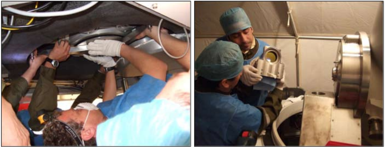
Figure 13-14. Photos taken during the replacement of the beam guiding prisms of the Coudé telescope. Upper left: Removal of a prism underneath the two-ton telescope. Upper right: Replacement of a prism mount.
