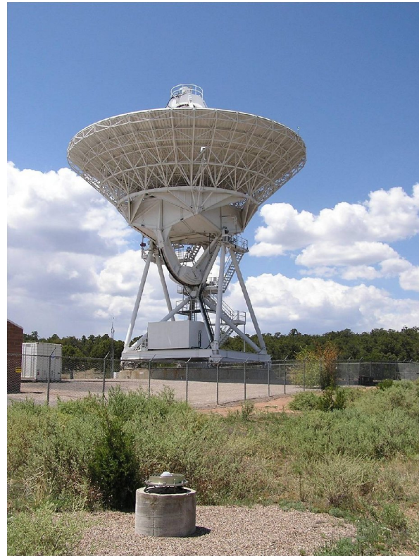
Figure 6 Pietown VLBA antenna with GPS antenna in foreground.
