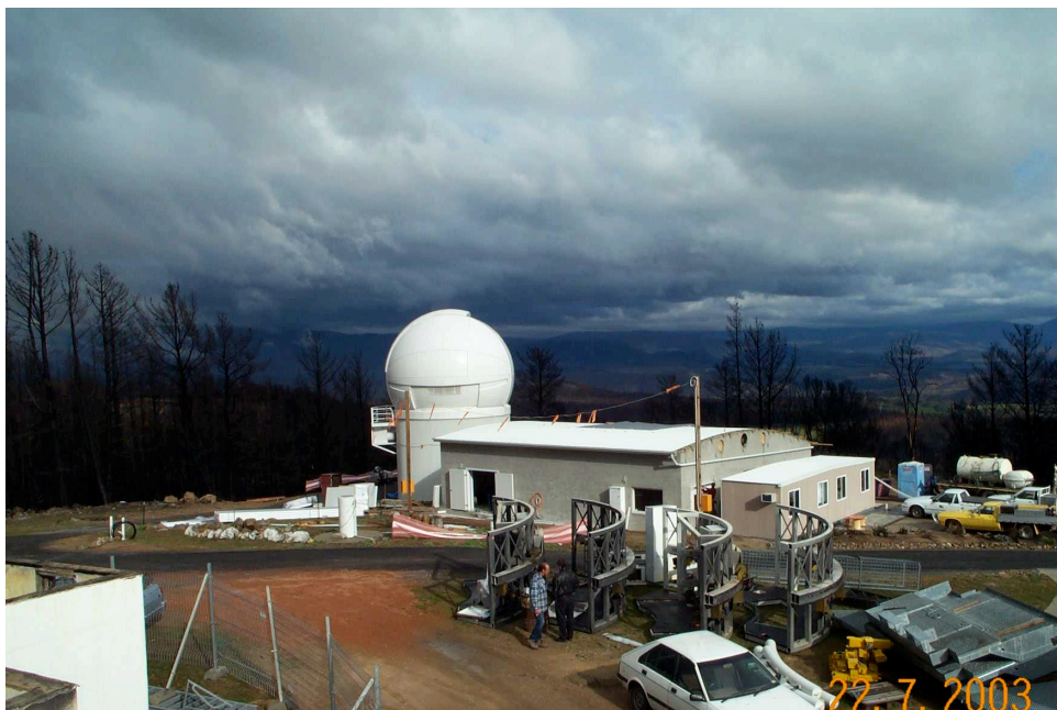
Figure 1b: The Stromlo site (July 2003) showing the SLR facility (prior to dome installation) and the 10m IceStorm dome housing the 180 cm telescope. Several telescopes are planned for the site.
