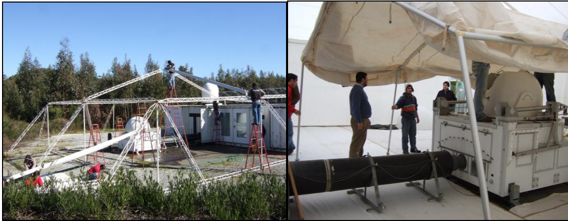
Figure 3. Construction of two interleaved tents to provide clean work conditions.
