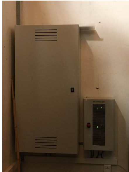
UPS 24VDC for SLR
